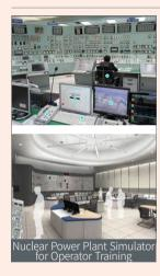
**Description** Nuclear Power Plant Simulator is to develop whole system, which are CORE, Thermal-Hydraulic, BOP(Balance Of Plant) and PPC(Plant Process Computer) system and Instructor Station, of the nuclear power plants for operator training. We, GNP SYSTEM, carrying out "Performance Test of the simulator" based on ANSI-3.5, 2009 that are Steady State Operation, Malfunction, Transient, Abnormal and Emergency Operation after the simulator development by ourselves
