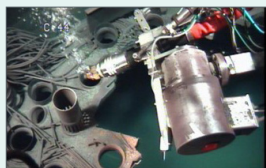
Dismantling and Decommissioning
