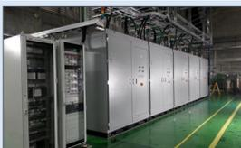
In-vessel Control Coil Power Supply
