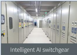
**Use** A power facility that receives extra-high voltage, converts it into high and low voltage, and distributes power stably to buildings and facilities
