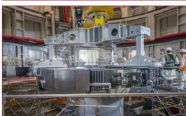
Central Column, CS Lifting Frame, PF Coil Supports
